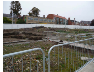
Hungate's new walkway
