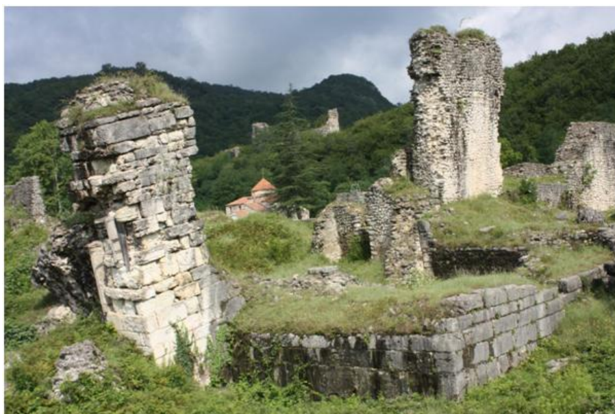
View of Nokalakevi. Forty Martyrs Church surrounded by imposing fortification walls (credit: author).
