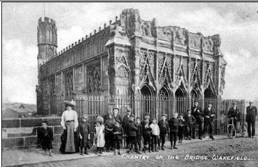
Figure 9. The Chapel between 1900-1910. The severe decay to the front is not evident on the previous photograph. Even if the photographs were taken 15 years apart the change seems very dramatic. (Anon. 1900-1910 [Photograph: Accession number: 1978.104/5] At http://www.wakefieldmuseumcollections.org.uk ). Image courtesy of Wakefield Council.
