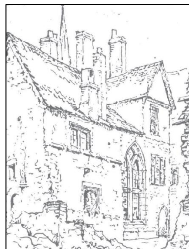
Figure 7. Buckler's sketch of the South West aspect following demolition of the post-medieval wings (Munby 1979, 135).
